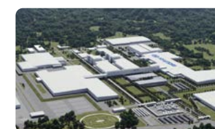
Plant #3 — Pune, Maharashtra
