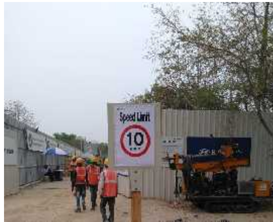
Figure 2.8. Workers using PPEs and signage for speed limits
