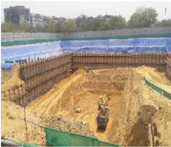
Figure 2.1. Showing construction status
