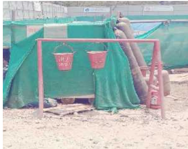
Figure 2.2. Fire Fighting Facility
