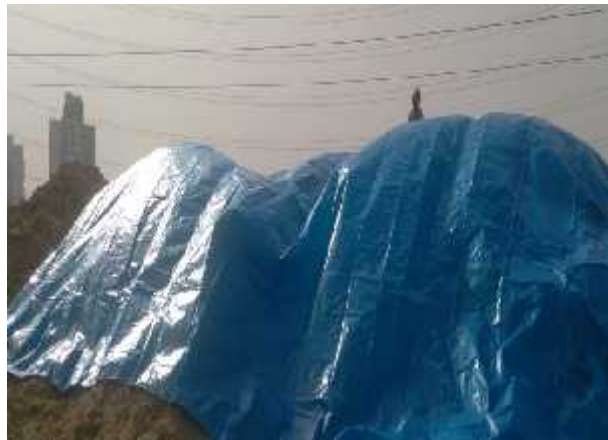
Figure 2.7. Covered Muck stored in the muck storage area
